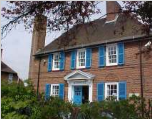
Northwood and Pinner Community Hospital
